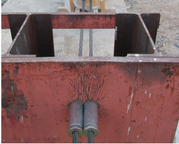
Figure 3.4 – Anchor prestressing strand using chucks (dead end).
