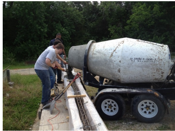
Figure 3.7 – Casting concrete.
