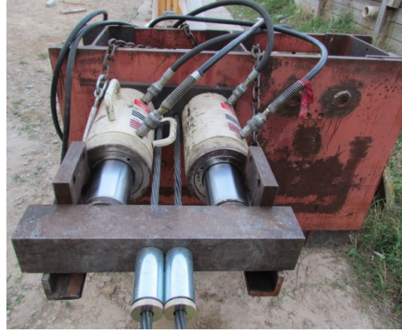
Figure 3.5 – Tension prestressing strands using hydraulic actuator (live end).
